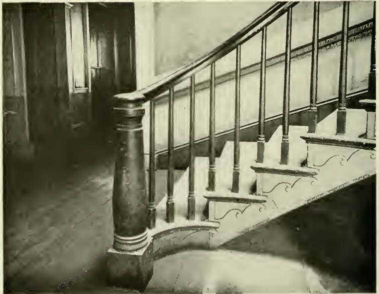
PLATE XLVII.—Stairway at Second Floor Level, Derby-Crowninshield-Rogers House; Detail of Newel and Stair Ends.
